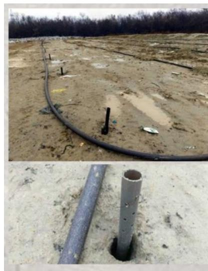
**Figure 7.** A line for collecting biogas
