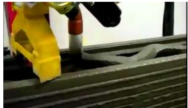
Fig. 1. Rising of a wall by extrusion of a concrete mixture from an operating nozzle on top of a previously extruded layer
