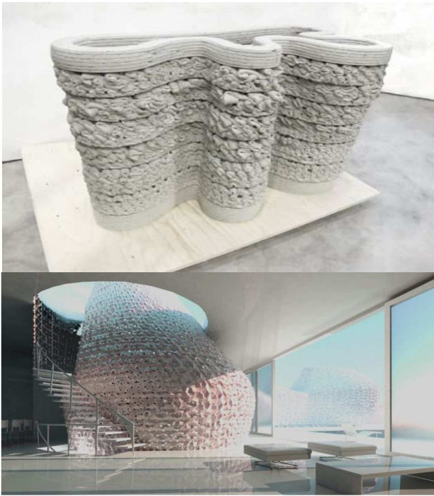
Fig. 1. An example of creative 3D printing application in construction industry [4]
